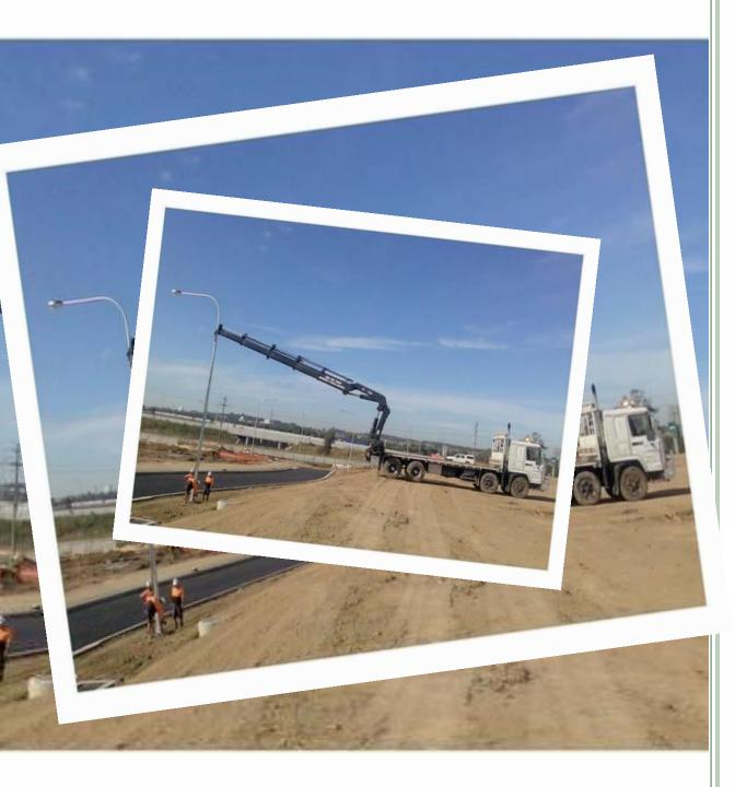
Cranetruck- 380 hp eight wheeler crane truck combination with a Hiab 36.60 (36 tonne / 1 metre rating)
